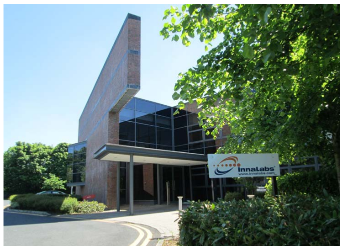
Figure 1. Innalabs Ltd Headquarter – 5,700 m 2 .
